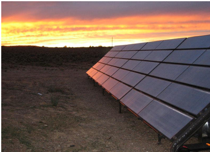
The solar thermal system above is capable of producing 800,000 Btu/Day equal to over 200 kWh/day of Thermal (heat) Power.
